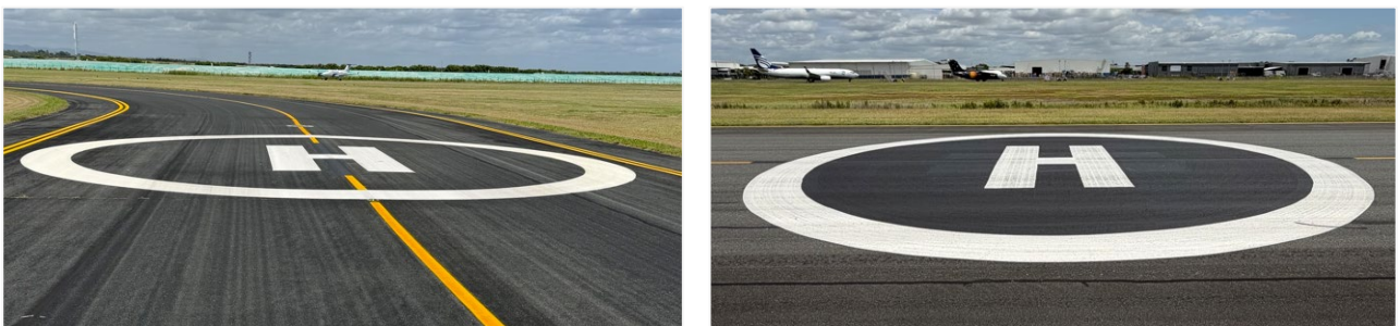
Figure 63 TWY F1 (left) and TWY L (right)
