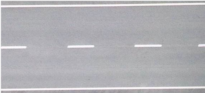
Figure 14 Perimeter Road Markings
