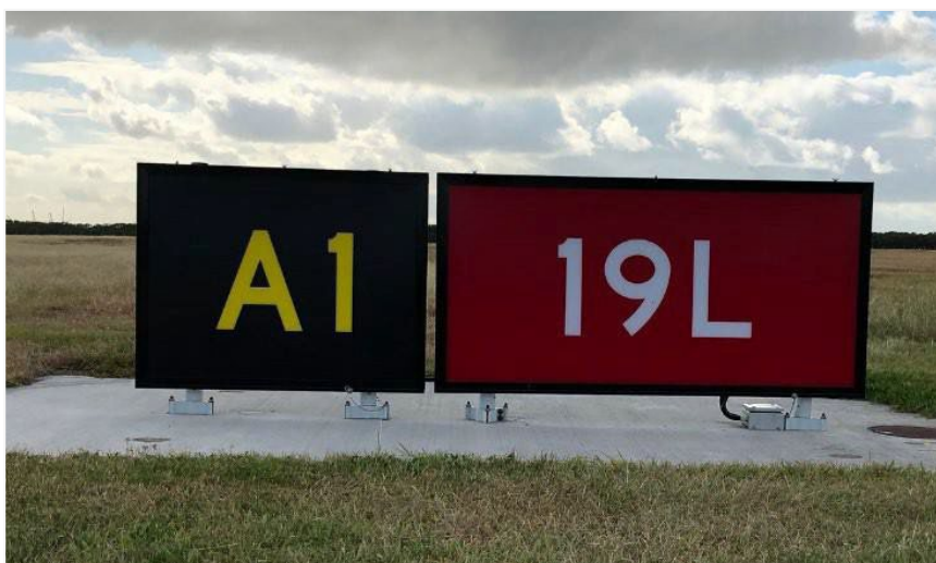
Figure 65 Runway Designation Sign
