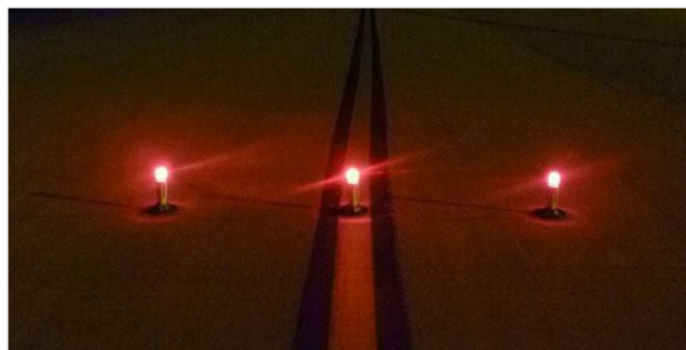
Figure 33 Red Steady Lights Replace U/S Cones at Night
