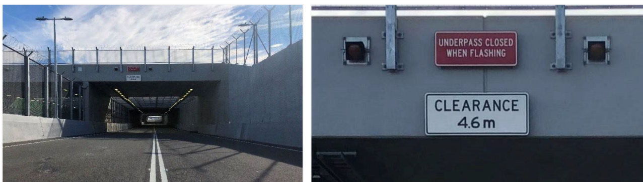
Figure 1 Dryandra Road Underpass Height Restriction
