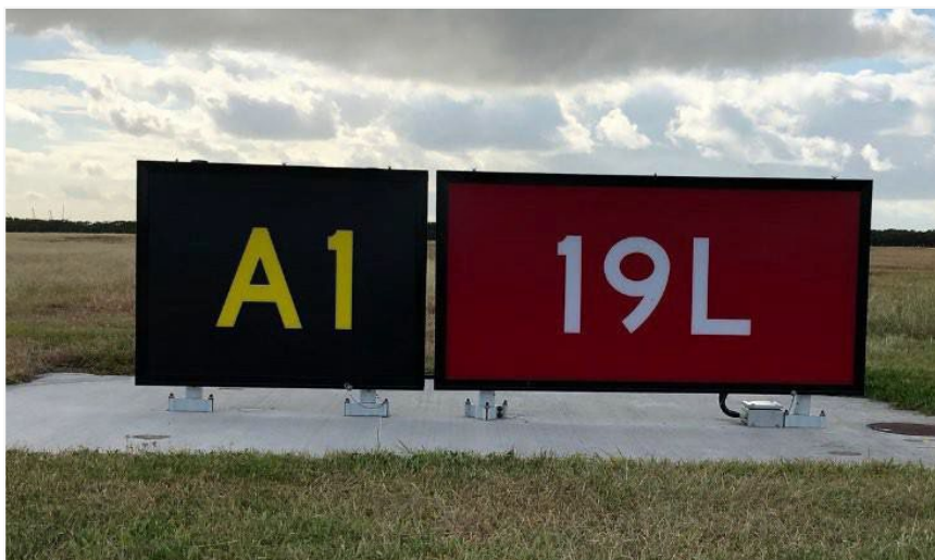
Figure 65 Runway Designation Sign
