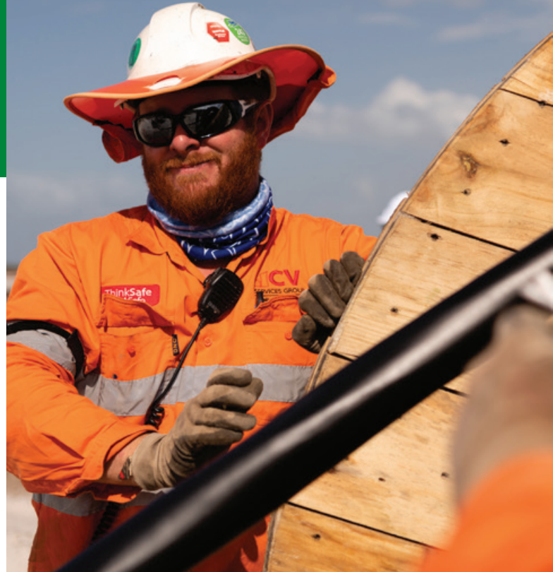
Installation of cabling on the new runway site. In total, 300km of cabling will be installed
