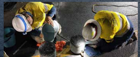
Installation of the Stop Bar lighting
