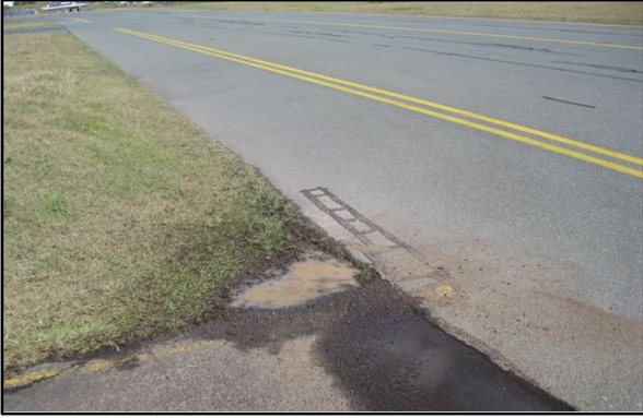
Figure 29 Example of leaving paved areas resulting in mud, grass gravel onto taxiway
