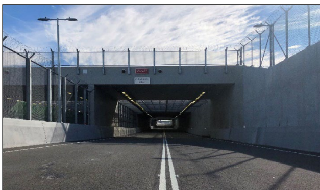
Figure 1 Dryandra Road Underpass Height Restriction
