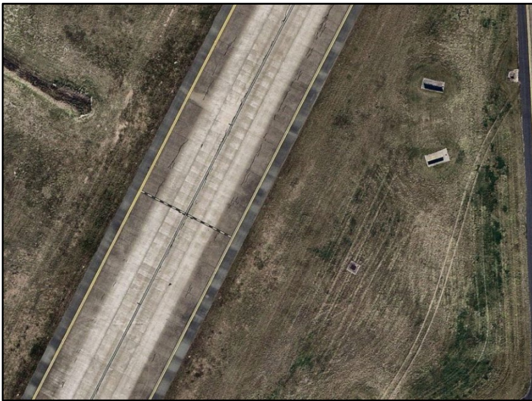
Figure 55 Intermediate Holding Point
