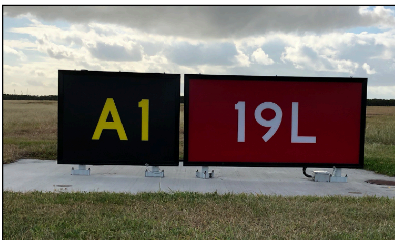
Figure 56 Runway Designation Sign
