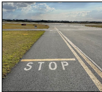
Figure 51 Warning Stop Sign and Stop Pavement Marking – Taxiway Mike looking toward RWY 01R-19L
