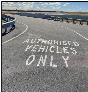
Figure 30 Authorised Vehicles Pavement Marking
