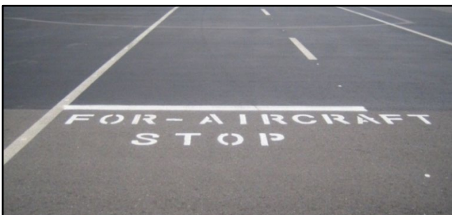
Figure 15 Stop for Aircraft Marking
