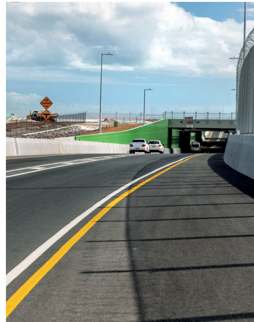
Dryandra Road Underpass
