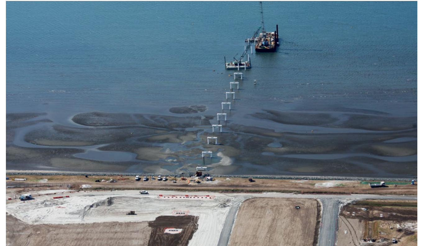
Installation of new Runway Lighting
