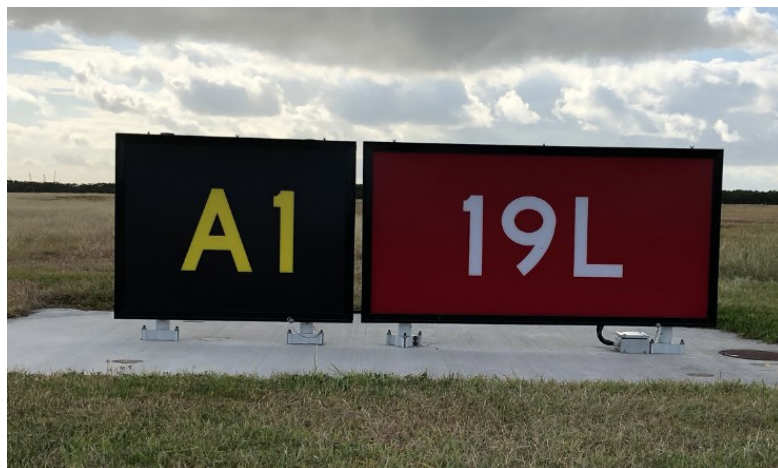
Figure 52 Runway Designation Sign
