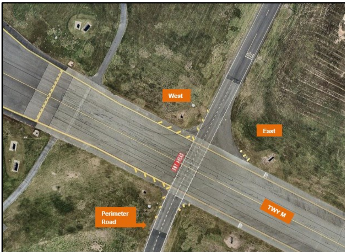
Figure 40 – Taxiway Mike / Perimeter Rd
