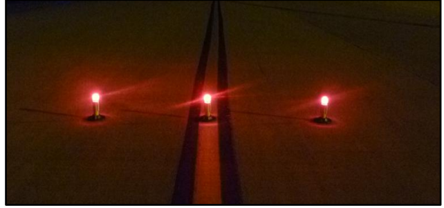
Figure 51 Red Steady lights replace U/S Cones at night
