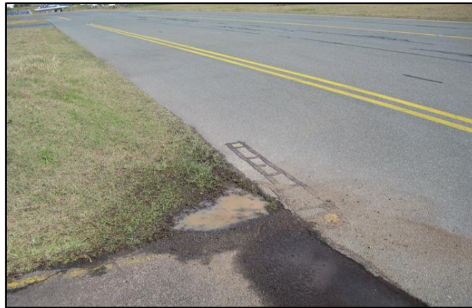
Figure 30 Example of leaving paved areas resulting in mud, grass gravel onto taxiway
