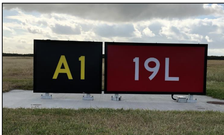
Figure 55 Runway Designation Sign
