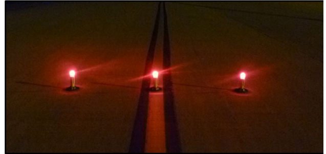
Figure 50 Red Steady lights replace U/S Cones at night
