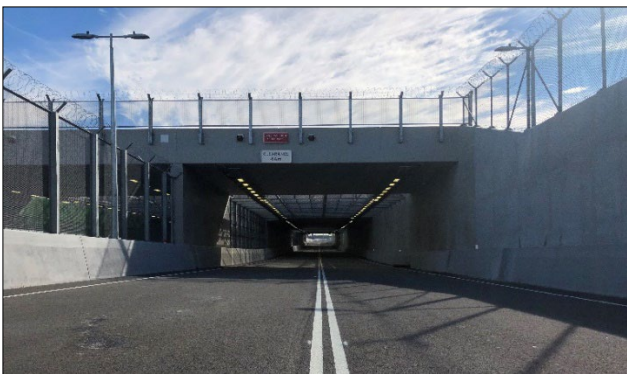
Figure 1 Dryandra Road Underpass Height Restriction
