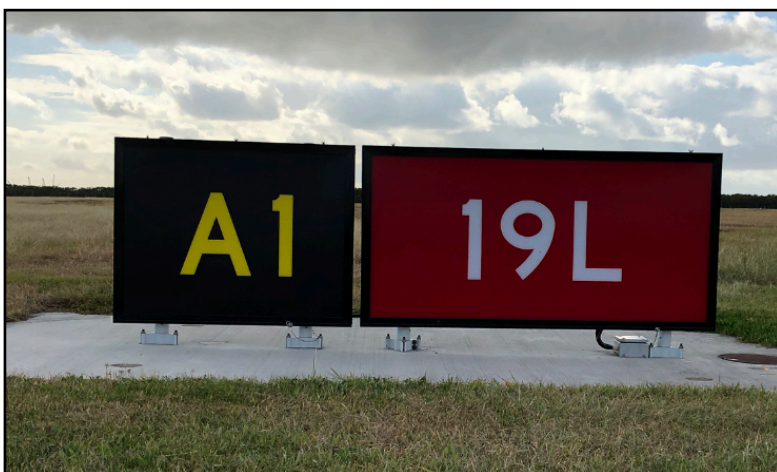
Figure 56 Runway Designation Sign
