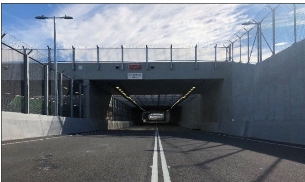
Figure 1 Dryandra Road Underpass Height Restriction
